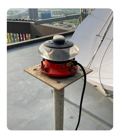
The apartment building was also fitted with one AV-OL-MI FAA L864 Medium Intensity Obstruction light at the highest point of the building. The Avlite Medium Intensity LED obstruction light is certified to the FAA L-864. LED obstruction lighting offer an ultra-bright, energy-efficient and cost-effective lighting solution.
