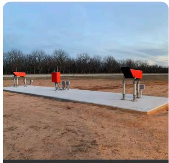
The Series 3 PAPI is Intertek certified to FAA AC 150/5345-28H. Patented LED technology provides the highest intensity, sharpest red/white transition line, and lowest power consumption.
