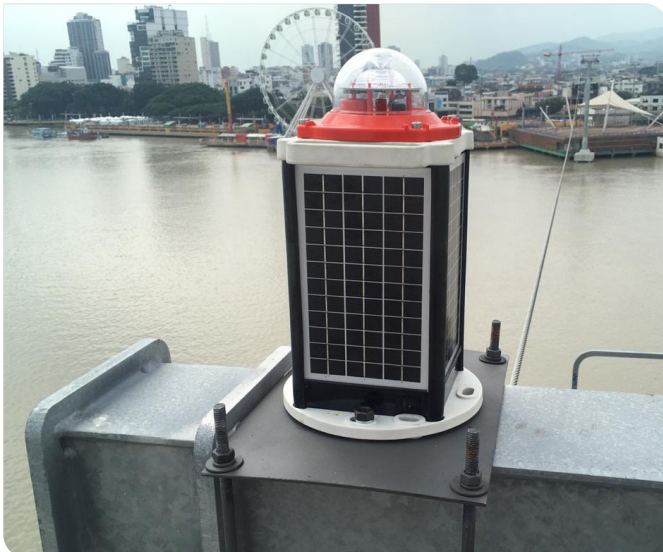
The AV-OL-C310 warns helicopters en route to hospital of a potential navigation hazard.
