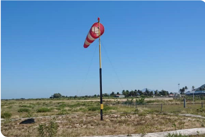
Internally lit L-807 Wind Cones provide surface wind direction to approaching aircraft.
