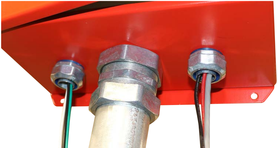
AC Connection Wires From PCU
