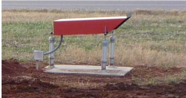
Example Of An Installed LHA
