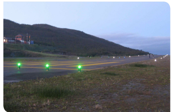
AV-426 solar LED Threshold and Runway Lights mark remote airfield.
