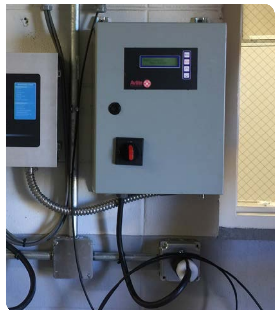
The Airfield Lighting Control and Monitoring System allows Avlite’s L-863 AV-70 Solar Taxiway Lights to operate as part of MCO’s existing airfield lighting system.
