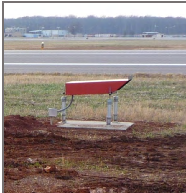
Example of an Installed LHA
