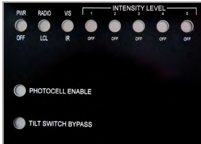
Power Control Unit (PCU) Control Panel
