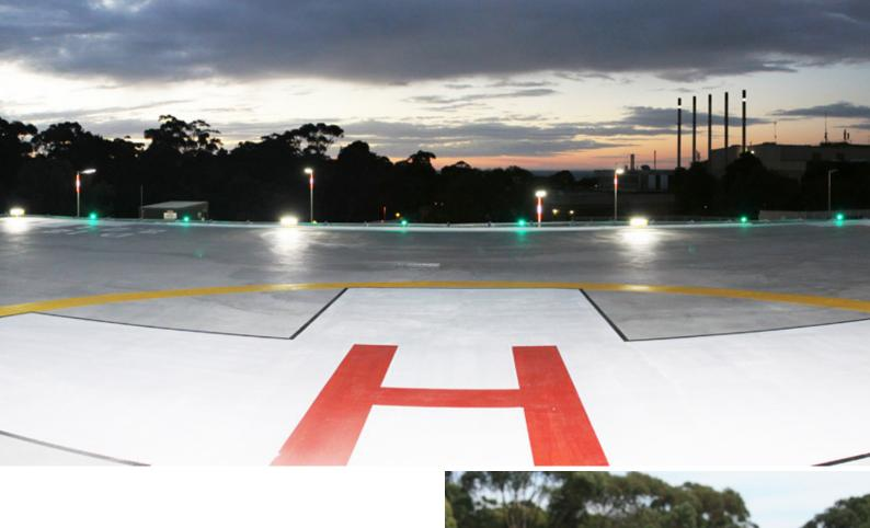
"The flood light demonstration illustrated the very neat tilt-adjustment feature that allows fine-tuning of the luminaire to provide the best light-spread across the heli deck without dazzling pilots upon approach," he added. "Since the luminaire is LED driven – with a life of up to 100,000 hours – our client will never need to worry about changing a light globe, ensuring this reliable, low-maintenance fixture has a low cost of ownership over its lifetime," Mr Simpson said.
