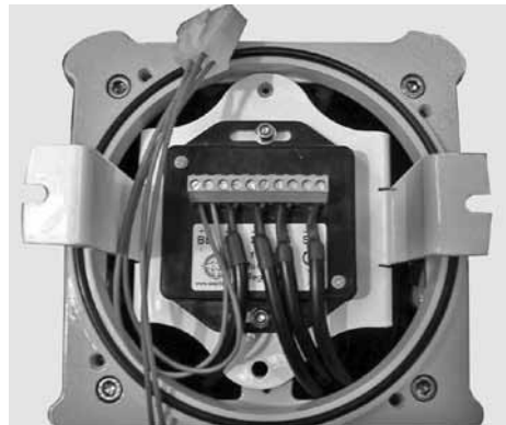
SL10 AMP Regulator shown when correctly fitted
