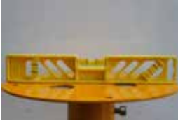
Check the mounting plate with a spirit level in all directions
