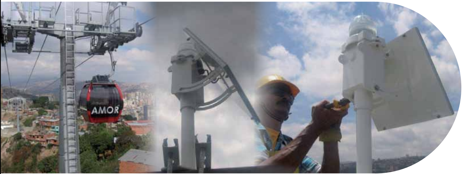
Images courtesy of Enersolar Ingenieria
