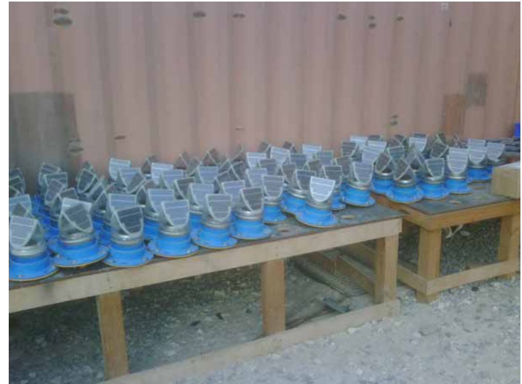
Taxiway lights getting ready for installation at an undisclosed air base in the Middle East
